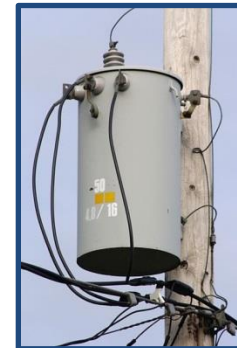
Singlephase polemount transformer steps the voltage down from the high voltage used in transmission line to 120/240 volts used in homes
